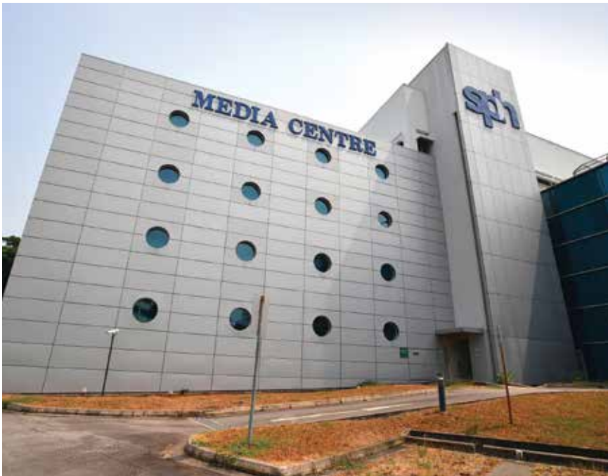
SPH entered into a JV with Keppel Data Centres Holding to jointly develop and operate data centre facilities at 82 Genting Lane
